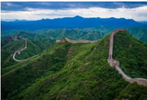
The Great Wall of China
